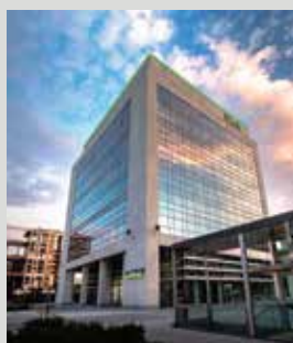
HQ Mansion of DKV, Spain
