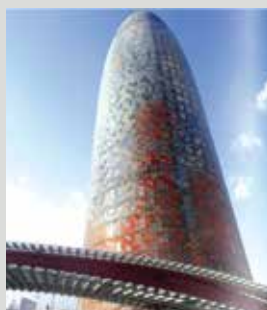
Torre Agbar, Barcelona, Spain
